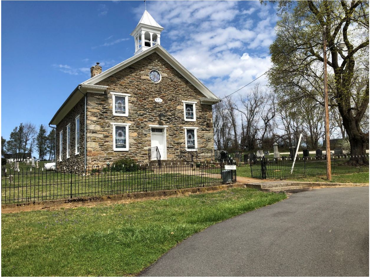
Historic Mt Olivet United Methodist Church on Mountain Rd, founded 1880. It's in the path of the transmission line from Short Hill.
