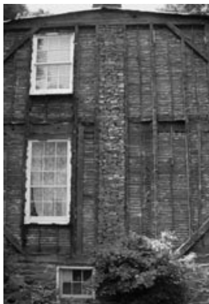
Balloon framing used in an 1861 Waterford house
