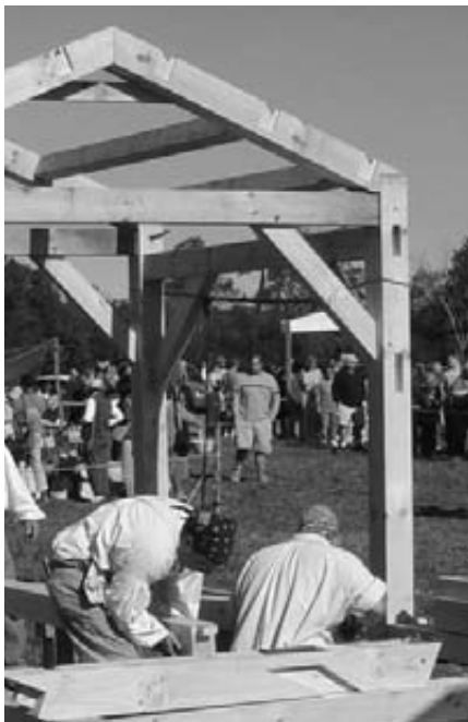
Demonstration of timber framing at the Schooley Barn area
